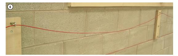
7a. Unscrew the eyehook from the Hexagon shaped Thimble and re-fit the eyehook by 3 turns of the thimble to ensure that the eyehook is secure.
