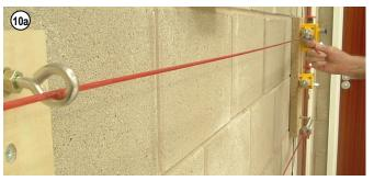
**11a.** Tension the system by holding the hexagon thimble whilst turning the switch eyebolt
