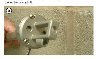
8a. Using the Allen Key (provided) open the locking bar in the main housing by
