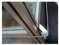
**4b.** For single switch systems, fit the QL to the Safety Spring.
